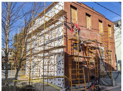
Repointing brick on front, installing stucco cladding system on side of building (EIFS-External Insulation and Finishing System. The first layer is foam board followed by a fiberglass mesh and a finishing coat.
