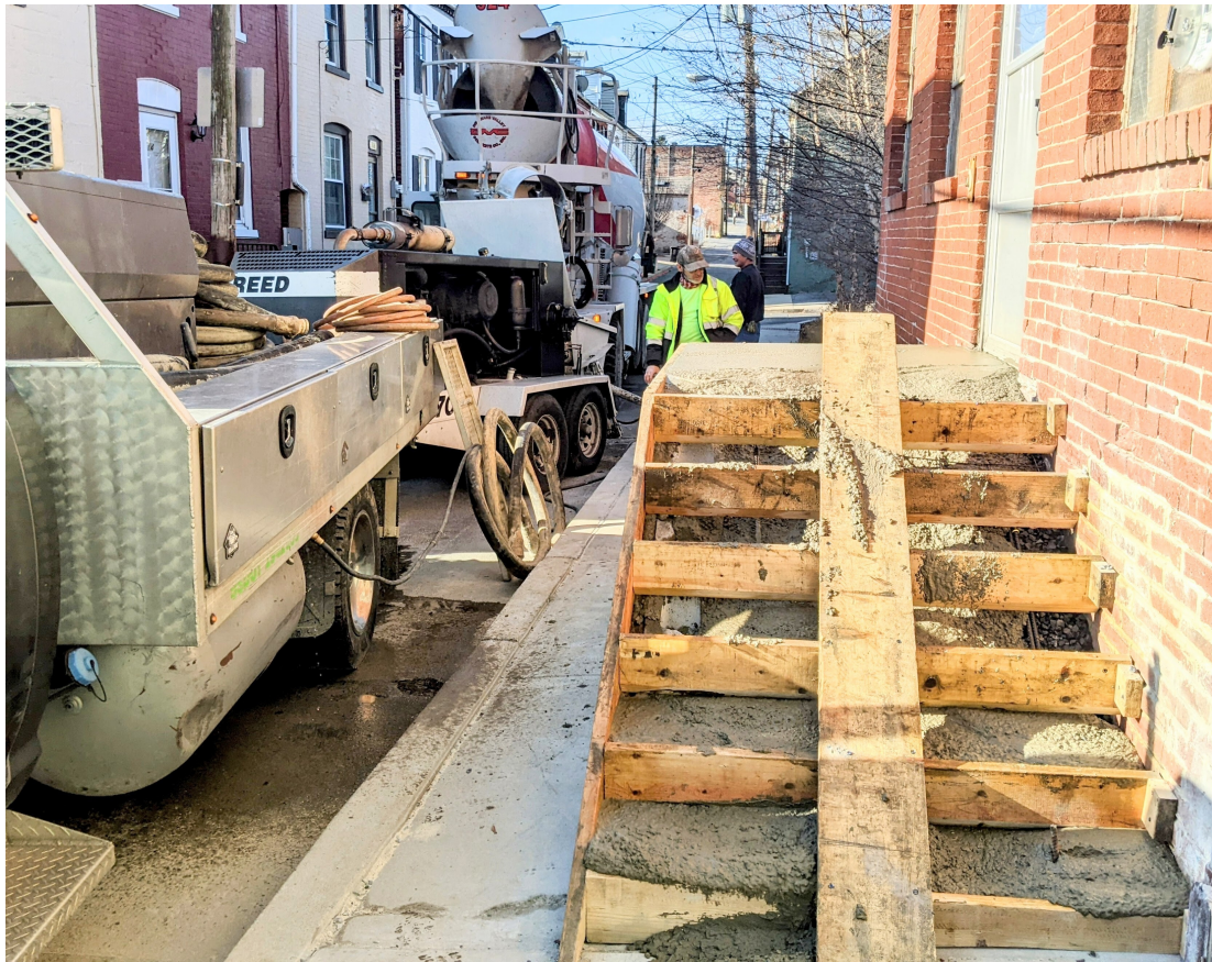
Pumping concrete for front steps on Grant Street and ramp access from parking lot.
