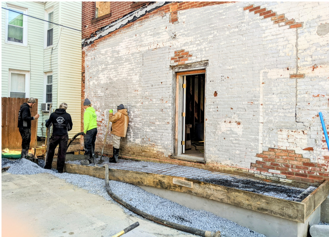
Pumping concrete for front steps on Grant Street and ramp access from parking lot.
